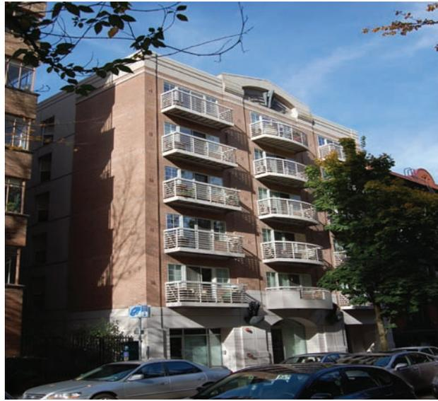
This six story infill project on Portland's South Park block needed to structurally deal with an adjacent building that was literally "leaning" over the property line. Rather than having the neighbor tear down the property, H & A worked with structural engineers to provide a structural system that could absorb the weight of the adjacent building during a seismic event. Construction sequencing was established that carefully avoided the out of plumb wall, avoiding further structural weakening.
