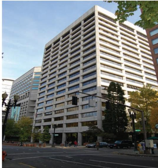
H & A has provided the Federal Government with full construction management on numerous projects at this 18 story building originally built in 1975. Upgrades have included numerous tenant remodels, and complete renovations of the mechanical system, fire alarm and elevators.
