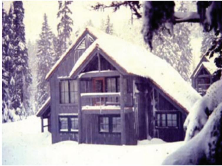
H & A provided full preconstruction services on this new 8 million dollar alpine facility located at Crater Lake. With snow loads (both vertical and lateral) in excess of 300#/square foot, careful consideration to every construction detail was paramount. The National Park facilities are located at an elevation of 8100' – only a scant three months of construction time is available per year.
